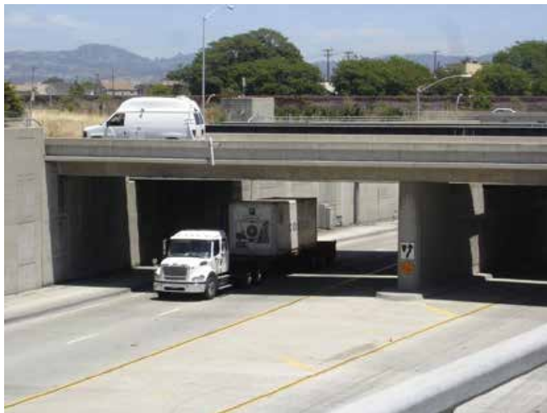
Figure 3.4 The Air District's mobile sampling van used to measure pollutant concentrations of exhaust plumes from Port trucks in West Oakland
